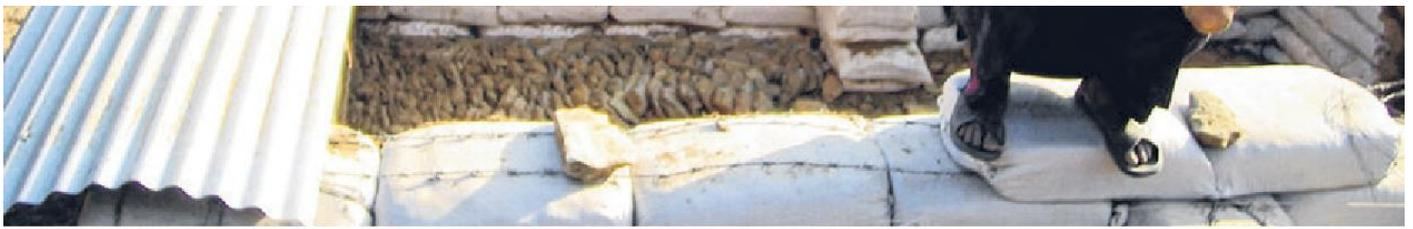
2. They are stacked on top of one another in a staggered fashion and held together by barbed wires. A trench is dug underground to form the foundation for the house.
