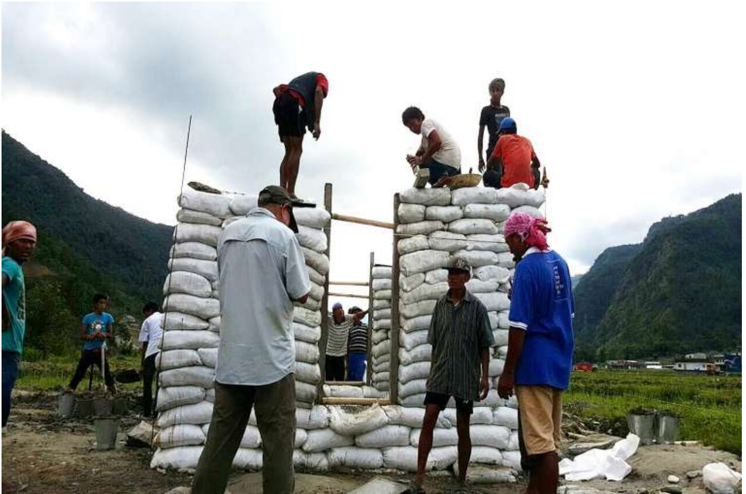
Nepalese building rice bag houses in a village near Pokhara. PHOTO: COURTESY OF KEE YI JAN, OPERATION HOPE FOUNDATION
